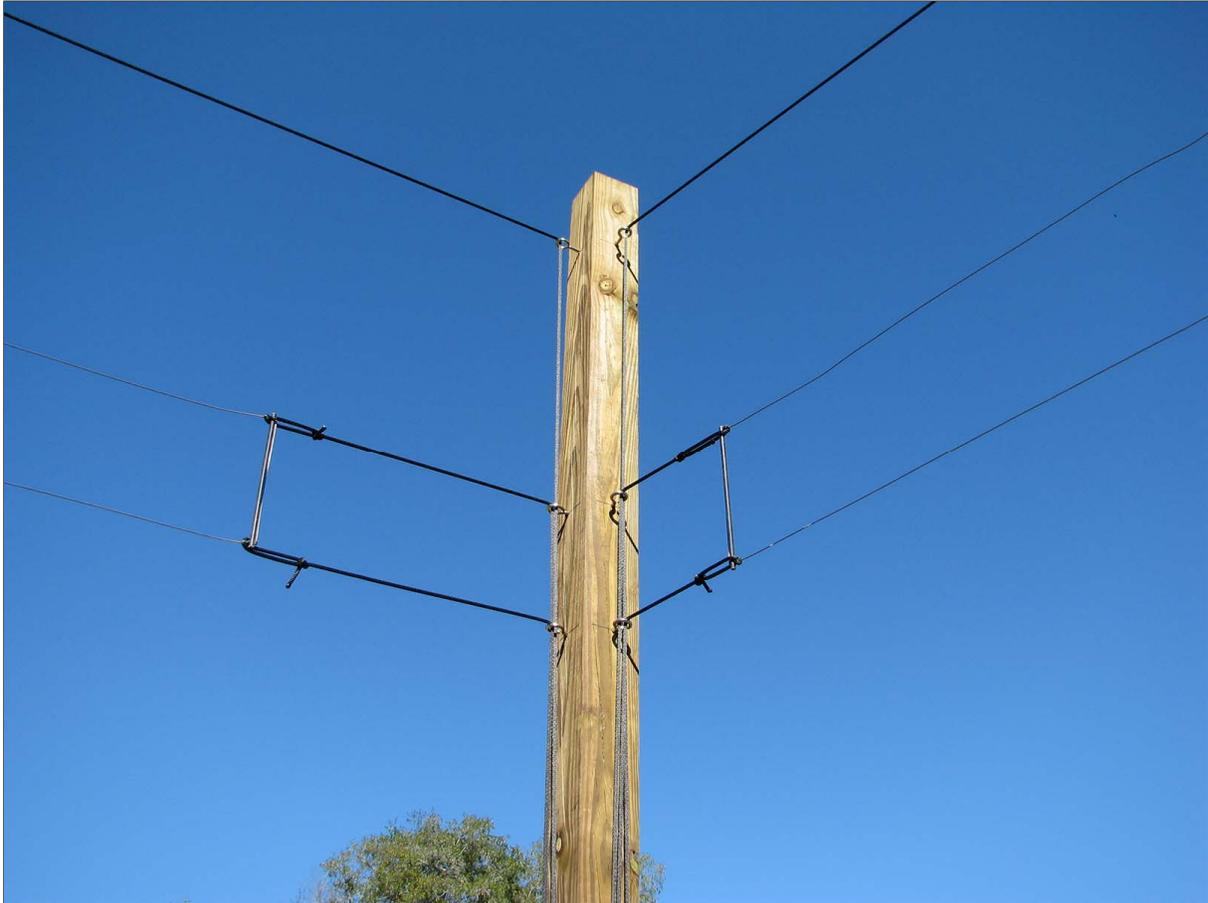
3/16" black polyester rope serve as halyards, running through stainless steel screw eyes. There is about 500' of rope in the array.
