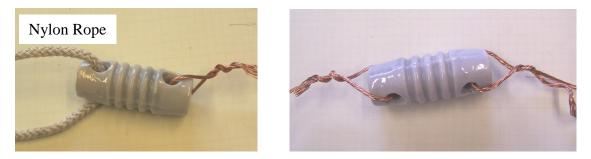
Figure 5.1a and 5.1b. Wrap the center and end insulators with the antenna wire.
