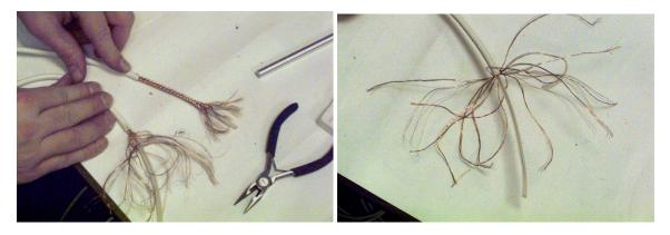
Figure 5.2a and 5.2b. Unbraid the copper shielding.
