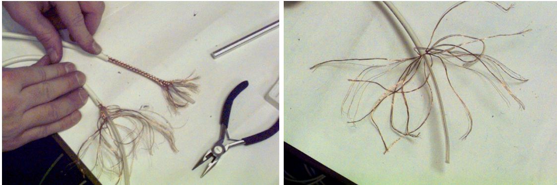
Figure 5.2a and 5.2b – Unbraid the copper shielding.
