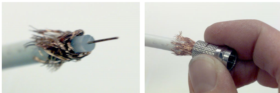
Figure 5.6d and 5.6e – Prepare the coax and install the F-connector.
